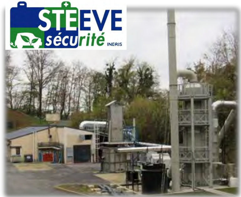
INERIS battery safety tests platform
